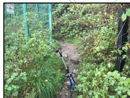
Currently there are no access controls at this point of the path. Access is limited however due to level changes and widths being tight between the existing fencing and the overgrown shrubs.
