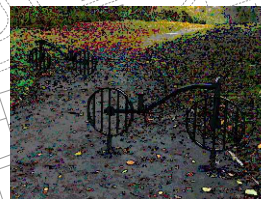
Proposed new horse friendly stile and new chicane barrier - TMBC standard detail M206
