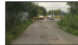
Current access control is a manual swing gate. When shut users are expected to walk around the post which is approximately 0.8m wide with a small embankment to the side.
